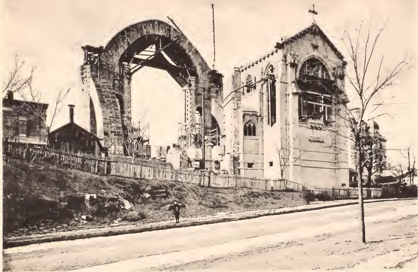
Cathedral of St. John the Divine. P. E. (in construction)
